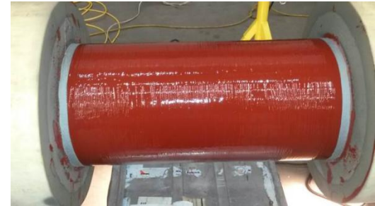
APPLIED 1 st COAT 300MIC
